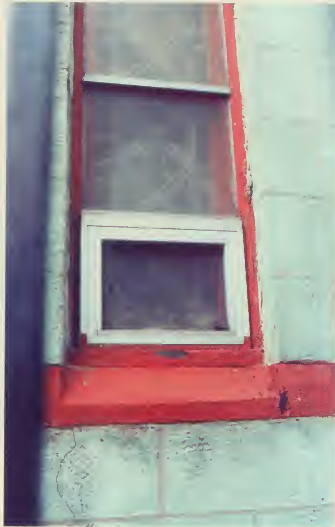
South Elevation of Church Building (T)
